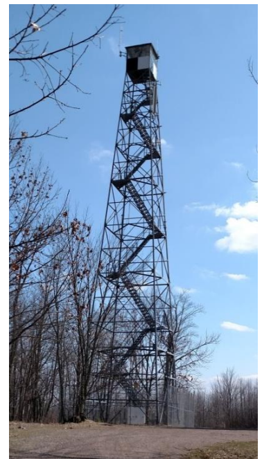
Connors Lake Fire Tower April 2016
